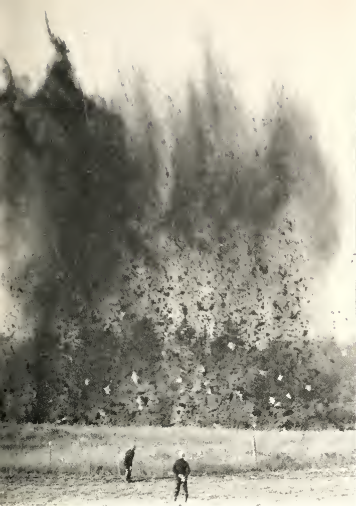
Members of the F.F.A. learn to apply the latest developments on their home farms. Here we see them using dynamite to make a drainage ditch on a school farm.
